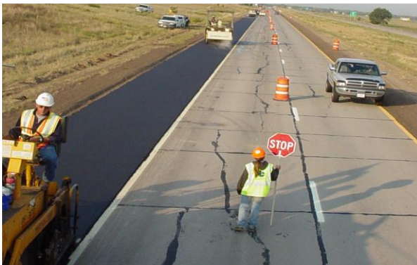
Region 4 Fort Morgan overlay project.
