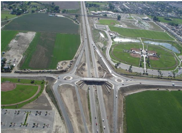
Region 3 I-70 at 24 Road Grand Junction. New bridge and two roundabouts
