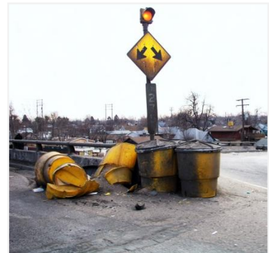
Impacted crash barrels at I-70 and York Street off-ramp resulting from inadequate deceleration lane length
