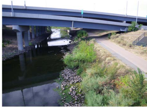
South Platte River intersecting with I-70
